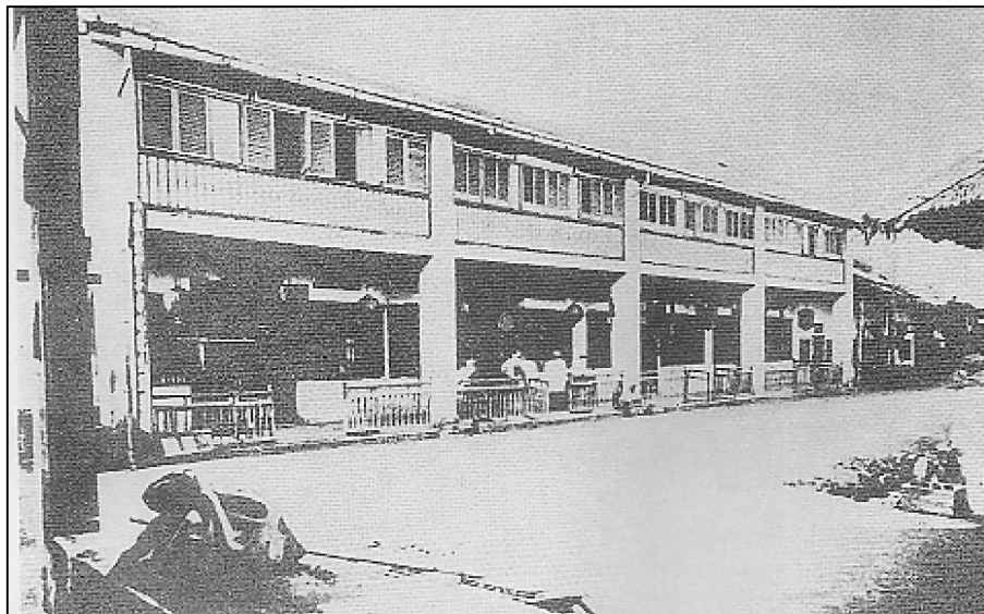
Figure 5: The first shophouses built in brick, sited in Old Market Square, and built by Yap Ah Loy, noticeably lacking the ornate fronts of later shophouses, though they are two-storey buildings of that type; Source: Gullick, J. M., (2000), A History of Kuala Lumpur 1856 – 1939, Selangor: MBRAS, p. 319
