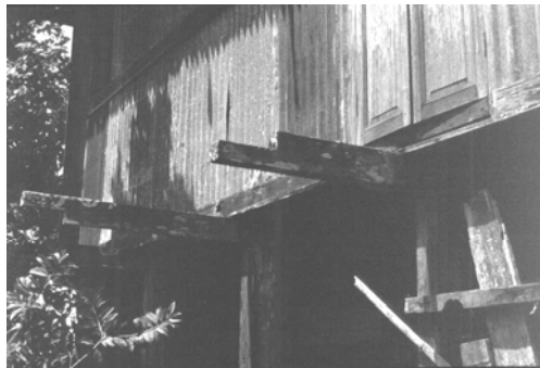
Fig. 10 – Floor beam projected out from Rumah Bujang indicates its connection with other parts of the house.
