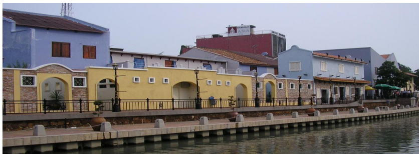
b: View from the river after upgrading
